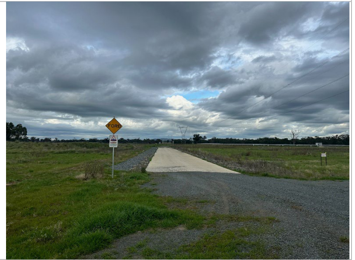
Photo 24: Permanent waterway crossing/drainage feature
