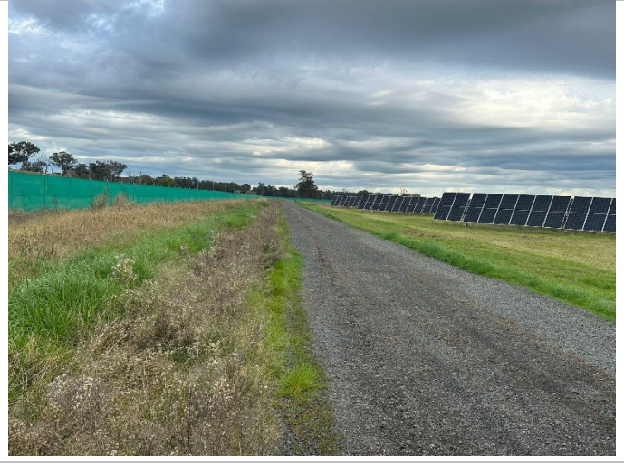
Photo 13: Sealed internal access road and weed die back
