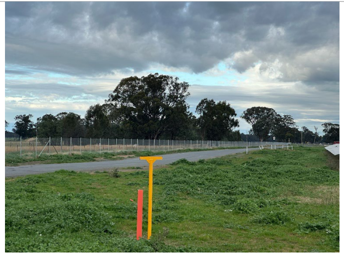
Photo 4: Location markers, APA high pressure gas main
