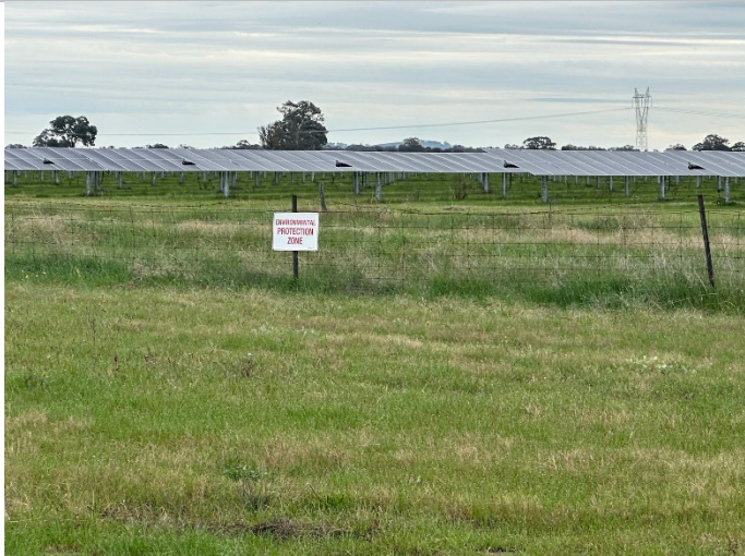
Photo 1: Solar panels and environmental protection signage
