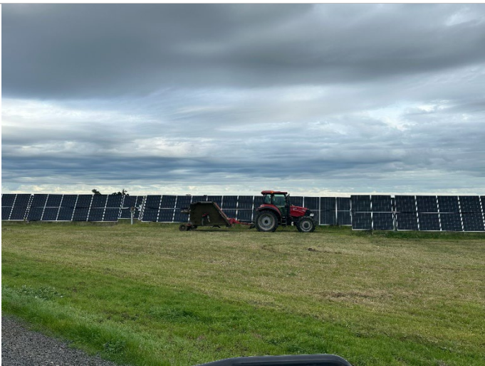
Photo 16: Slasher in operation
