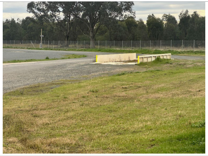
Photo 15: Construction phase rumble grid and vehicle washdown, retained for BESS construction
