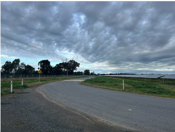
Photo 14: Sealed internal access road
