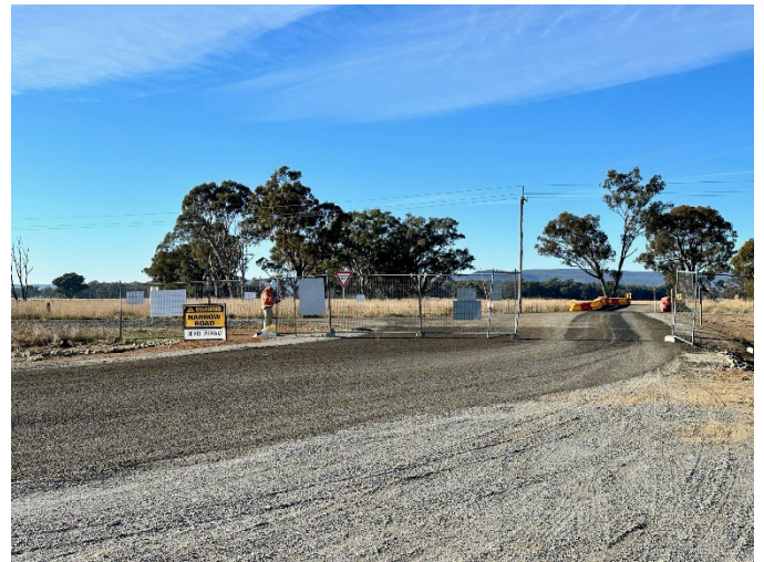
Photo 4: Stabilised site access
