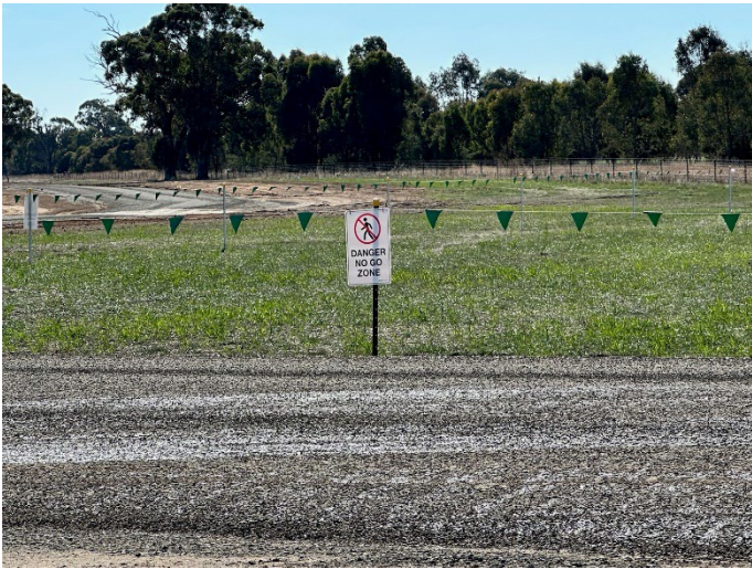
Photo 19: Restricted access, no go fencing and signage for APA zone
