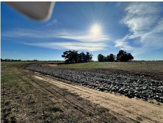
Photo 21: Temporary creek crossing, scour protection
