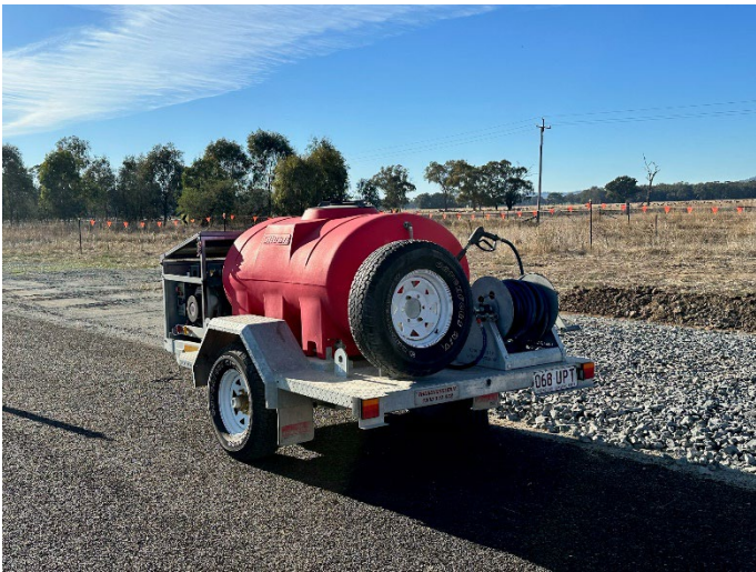
Photo 3: Temporary Vehicle washdown and rumble grid construction
