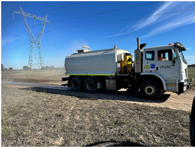
Photo 11: Watercart utilised for dust suppression
