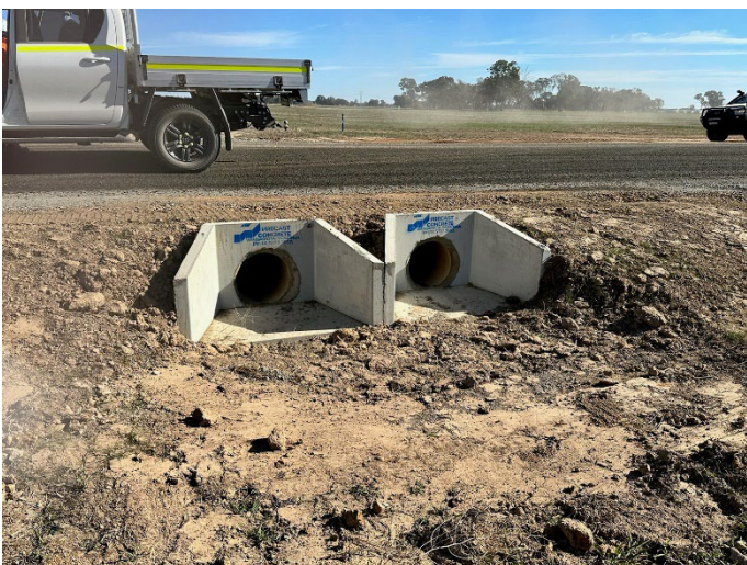
Photo 23: Drainage culverts, internal access road
