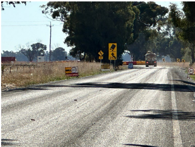
Photo 15: Completed road upgrade
