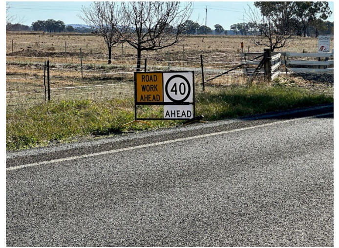
Photo 14: Speed restriction signage
